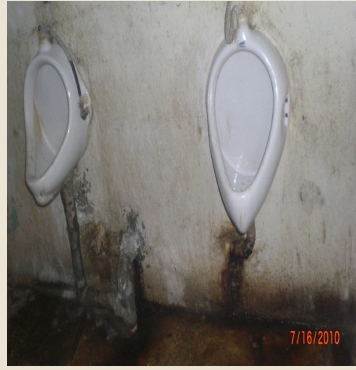
Current Photo of Boys Restroom
